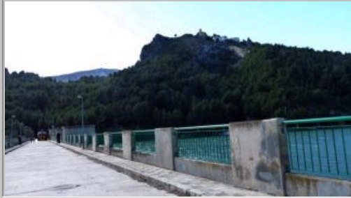
Staumauer N 38° 40' 50.5'' W 0° 11' 29.5''
